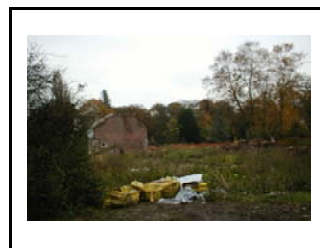
View looking across the site of the former Cottages.
