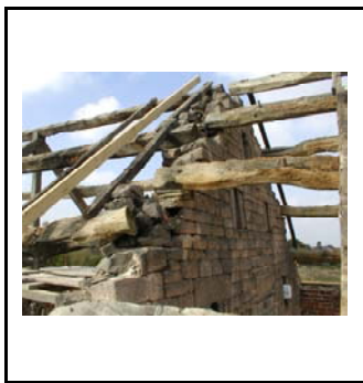
Exposed timbers on a historic barn.
