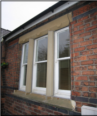
Sliding Sash Windows Traditional on Victorian Properties
